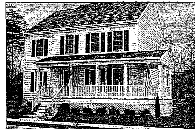
Variation can be achieved by shifting porches to the side to suggest, but not actually achieve, a wrap-around. Large informal porches that can serve as "outdoor rooms" are the hallmark of this style. The lack of a roof overhang on the gable end is inappropriate.
