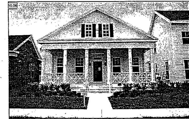
On a more modest home, attention to a few key details, such as shutters on the upper windows, and a classical balustrade, create an elegant appearing home within a classical design vocabulary. Traditional roof forms, such as simple hipped or gabled, allow more emphasis to be placed on the front facade and not on the roof mass.
