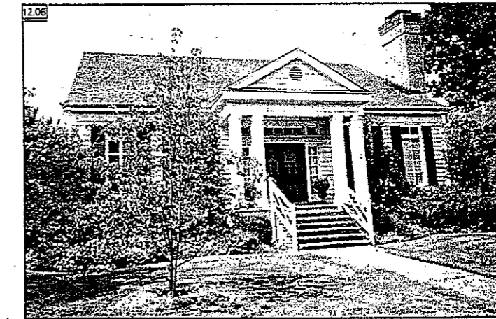
Use of a pediment and fenestration together with a raised porch and columns can add a feeling of importance to cottage-style homes.
