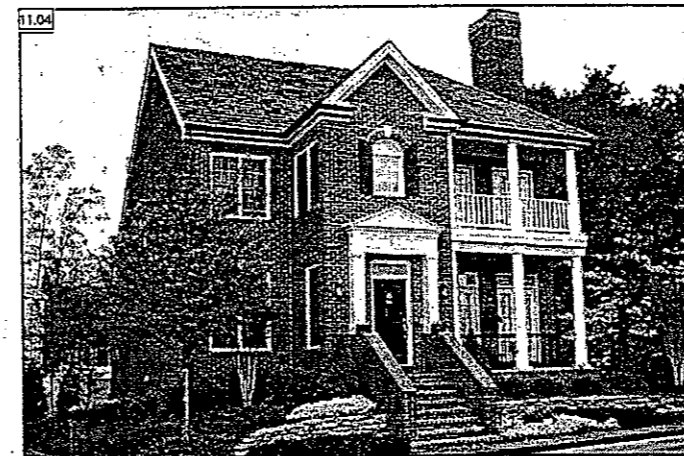
This Colonial-inspired reinterpretation pulls the entry bay forward to help inset the porch and balcony. The front entry detailing and stair could have been more appropriately detailed.
