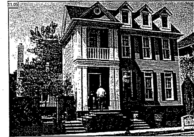
Paired columns, dormers, and tall, detailed windows create an accentuated vertical proportion to this house. The brick base, entry steps and raised foundation allow the house to sit closer to the sidewalk.
