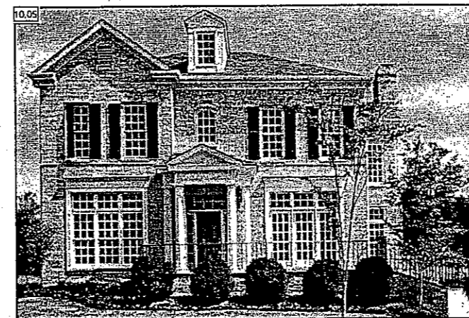
While breaking somewhat from the rules of pure style, this classically-inspired home successfully blends a gable into the facade composition. Window proportions and front entry detailing keep the house firmly within a classical design vocabulary.
