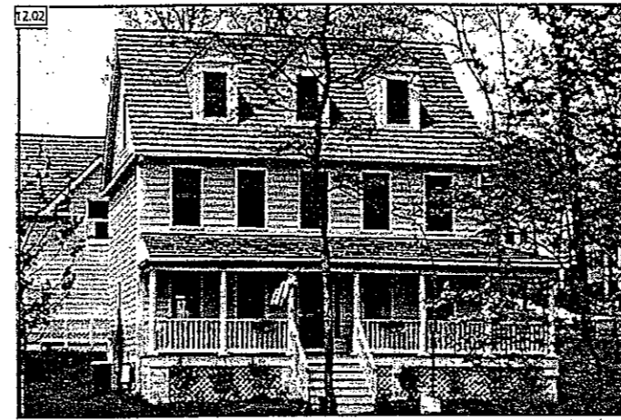
Finished first floor is raised above grade and accentuated by a porch with a lattice skirt. Dormers can further add to the vertical proportions of the simple mass.
