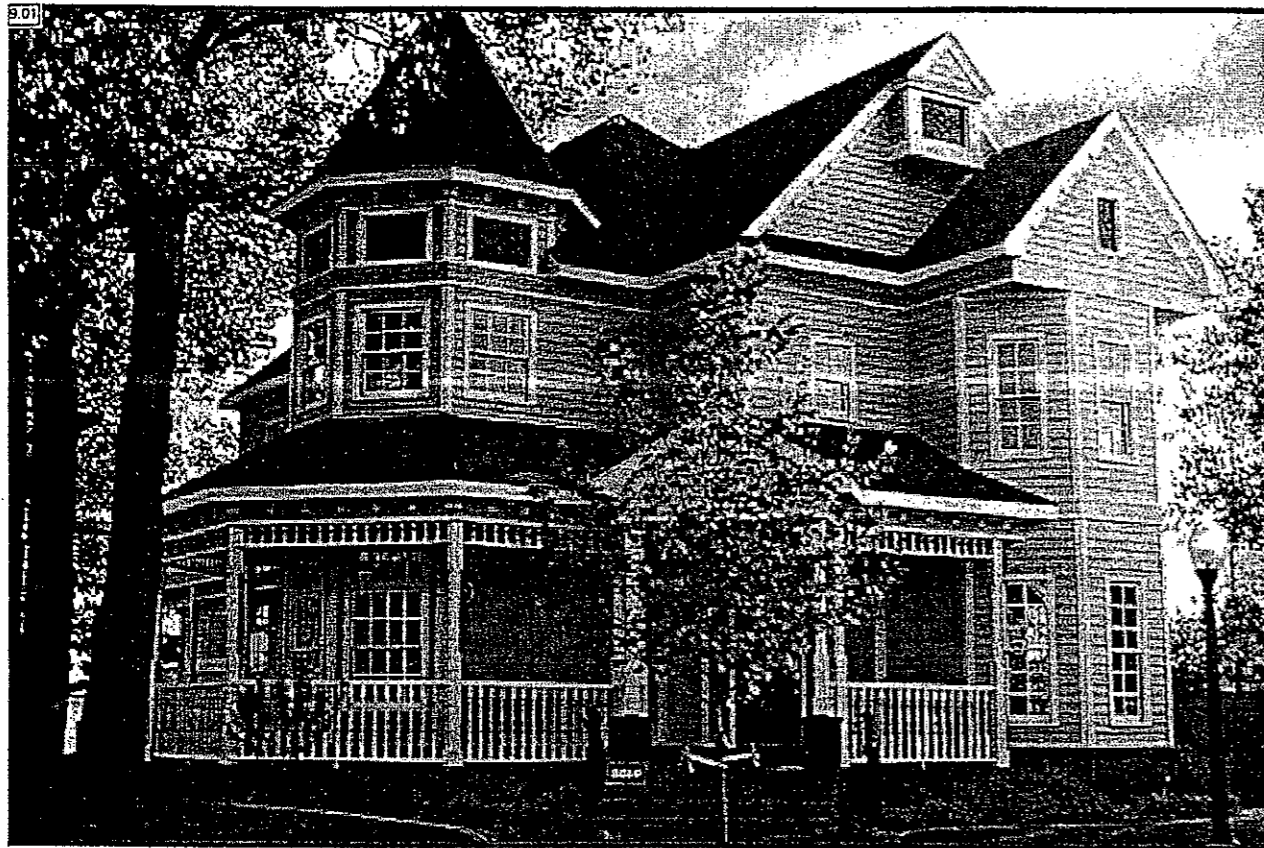
Asymmetrical massing, variety in roofline and projecting bay windows are the basic form of Queen Anne-inspired Victorians. The turret, together with a wrap-around porch, creates a strong corner treatment.
