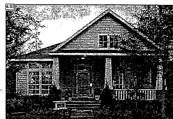
Craftsman and cottage style homes with a front projecting gable lend themselves to the footprint and massing of the forward bay porch (see V-6 above). The single offset to the main body in this form accentuates the porch while creating visual interest to the curb appeal of a smaller home. Research indicated that this house was highly popular.
