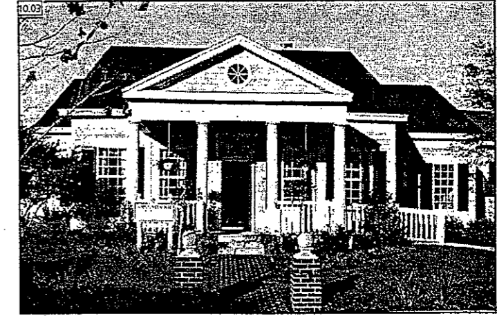
A well-proportioned porch framed by a series of columns provides a sense of formality and importance to single-story homes. Wings on both sides allow the floor plan to extend out in clearly punctuated steps that result in a highly interesting curb appeal in the front and defined patio spaces behind.
