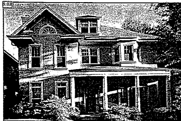
Plans with centered entries and symmetrical room arrangements can also be accommodated in a Victorian Revival form. The forward gable is counterbalanced by the inset front porch and projecting bay window.
