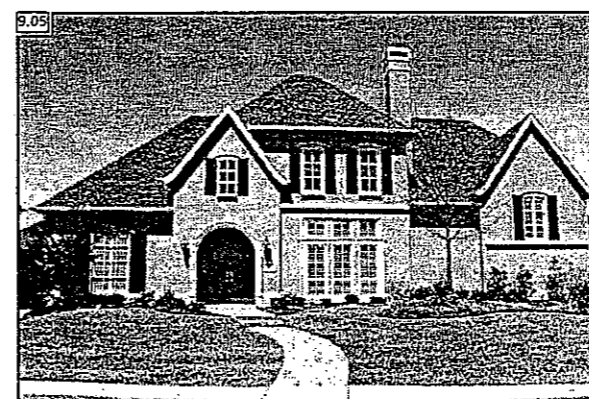
Projecting gables anchoring both ends of the house create appropriate balance. If the hipped roof on this house was gabled and some other details adjusted, this house would be more true to the original style.
