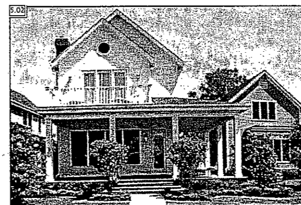
Wrap-around side porches with few balustrade details provide an open, welcoming image in relation to the street (see C-6 above). This type of porch is a hallmark of the Texana Farm-house style.
