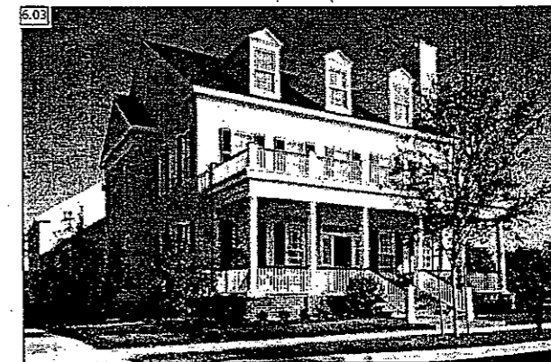
Example of a full front porch with projecting secondary gable to respond to corner location (see M-1 above).
